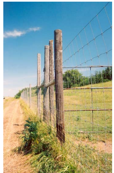
Poles taken out of service by Kandiyohi Power were recycled for corner post structures on this elk ranch north of Wilmar, MN.
