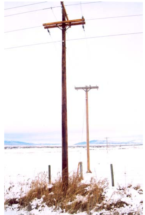
Southwest Montana is one of the few areas where high-grade talcum is mined. Expanding operations of a local mine required additional power. Vigilante Electric built a new three-phase line using 40 ft., Class 5 cedar poles along Sweetwater Road, above, and for the line to the mine, below. Talcum is not only used in powder, but it is also used in the paint and plastics industries.
