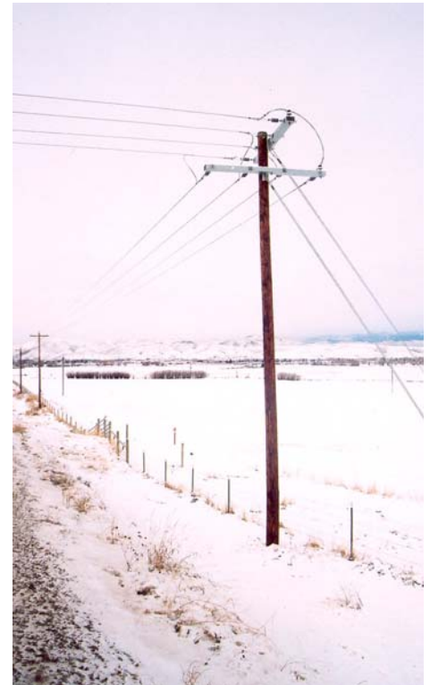
Southwest Montana is one of the few areas where high-grade talcum is mined. Expanding operations of a local mine required additional power. Vigilante Electric built a new three-phase line using 40 ft., Class 5 cedar poles along Sweetwater Road, above, and for the line to the mine, below. Talcum is not only used in powder, but it is also used in the paint and plastics industries.
