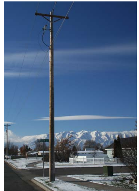
Above, part of the ongoing loop line conversion from 46kV to 138kV, poles were originally located on the opposite side of the street before this line was rebuilt. This double circuit 138kV line uses 75 ft. Class H-1 cedar poles. Below, a typical 12.5kV cedar distribution pole, this line uses 45ft. Class 4 poles.
