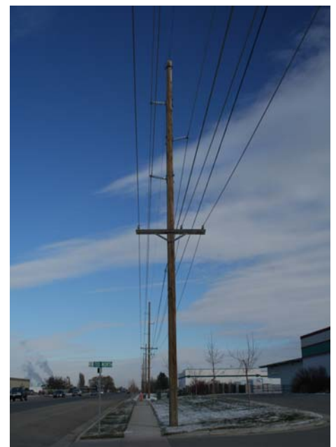
Above, part of the ongoing loop line conversion from 46kV to 138kV, poles were originally located on the opposite side of the street before this line was rebuilt. This double circuit 138kV line uses 75 ft. Class H-1 cedar poles. Below, a typical 12.5kV cedar distribution pole, this line uses 45ft. Class 4 poles.
