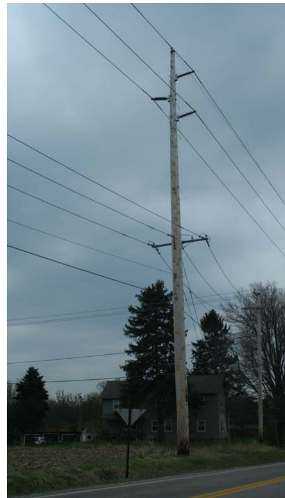
This street that crosses Interstate 75 uses 95 ft. H-2 Western Red Cedar poles and carries both 12.5kV distribution lines and 69kV transmission lines as part of the loop system around the city of Wadsworth.
