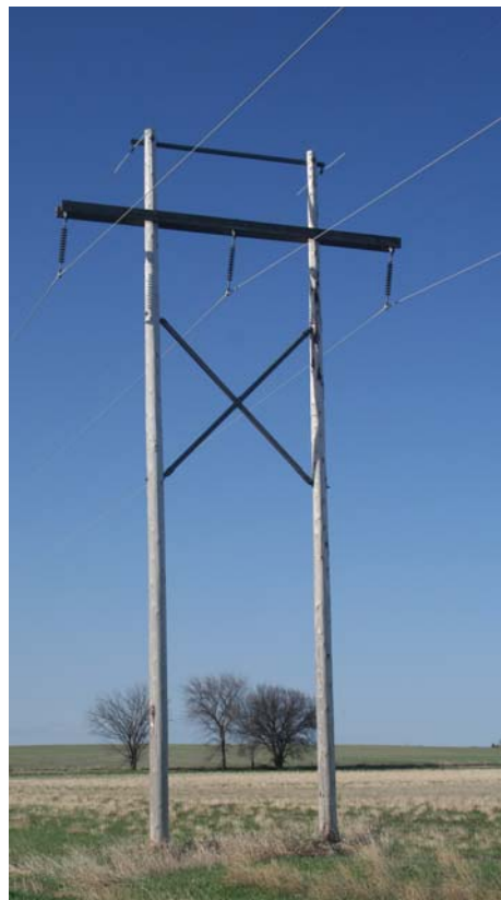
Rosebud Electric Coop uses Western Red Cedar like this 70 ft. transmission pole because of its durability, climbability and ease of handling.
